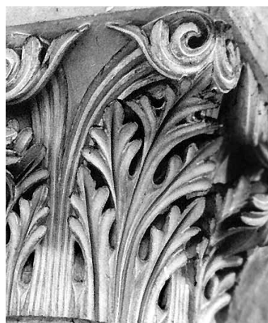
Laon aisle Ne2s(a) corner detail
